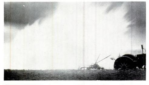
This fire was plowed up by a farmer's son named Walter Heck. Walter was driving his father's tractor across an alfalfa field when his plow sliced through a temporary gas pipeline. The gas, ignited by a spark when the steel plowshare struck the pipe, flared up, enveloped tractor and plow in a sheet of flames, singed the seat of the overalls of fleeing Walter Heck.
